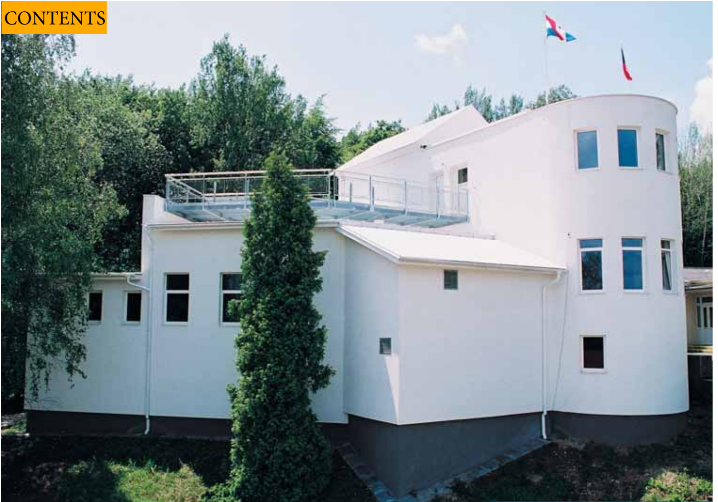
Observatory – building after reconstruction
